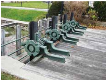
Gates at the mill race that can be raised to allow water to flow into the White River thereby controlling the level of the lake.
